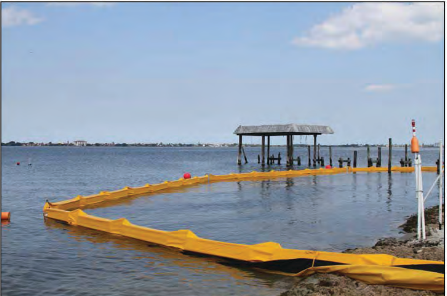
New turbidity curtain installed on site. Image courtesy of GEI Works.
