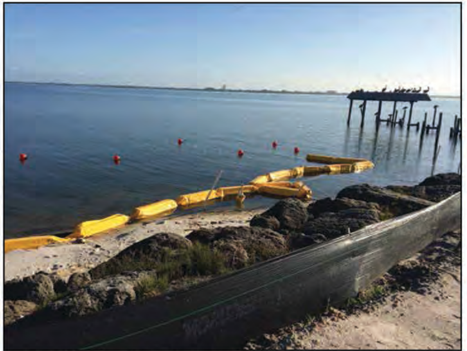
Above: Turbidity curtain out of position due to ineffective anchoring. Below: Installed T-posts failing to hold the curtain in place. Images courtesy of GEI Works.
