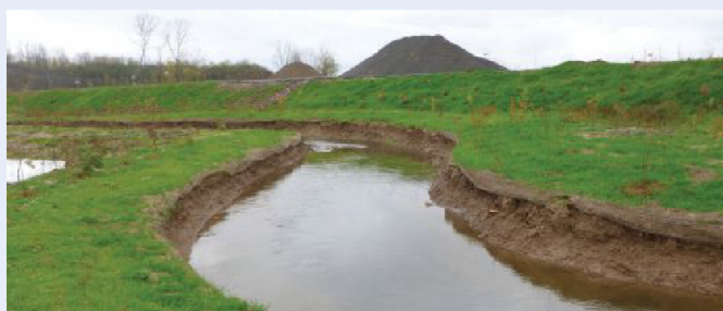
Vegetated re-growth over coir matting overlay at reclamation site in Super Fund Project tributary. Photo from the Parson's Geddes Brook Onondaga Wetlands Project
