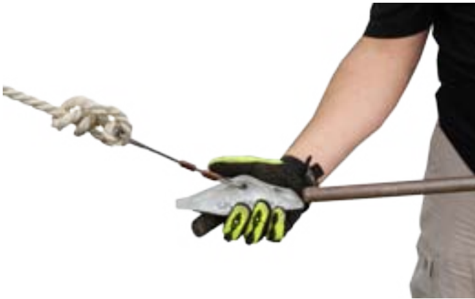
Step 5: Insert the driving rod into the existing hole in the anchor.
