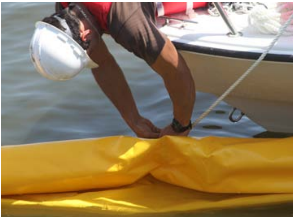
Step 10: Tie the rope to the anchor point on turbidity curtain.
