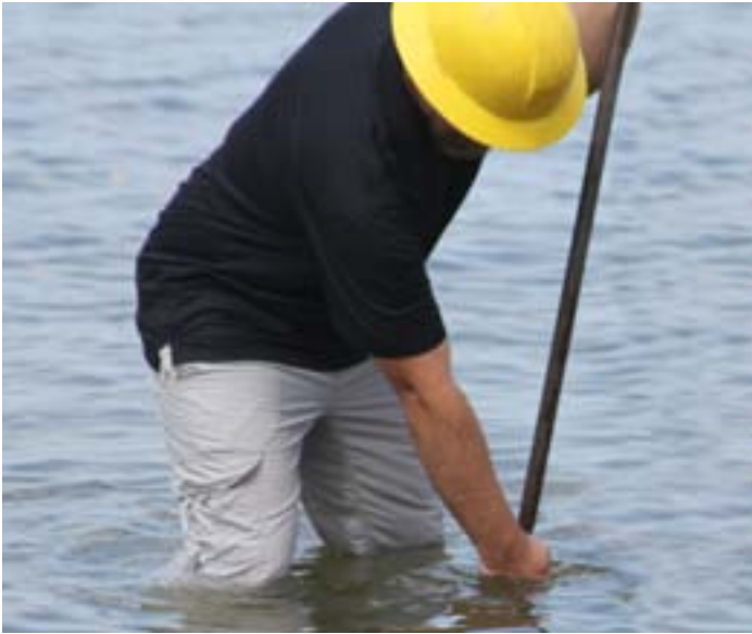
Step 8: Twist the rod so it loosens from the anchor. Pull out the rod once it is completely loose.
