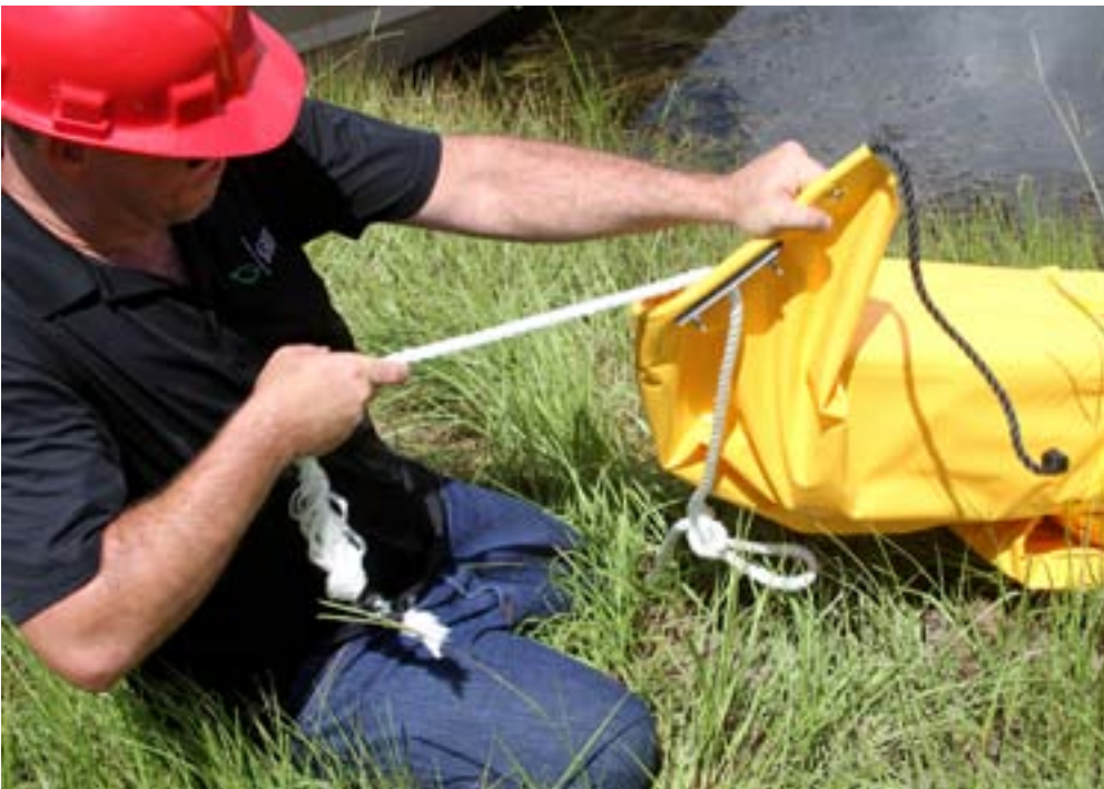
Step 7: Set the anchor for maximum loadlock by pulling vertically on the rope with a substantial amount of force. This will shift the anchor into position for full stability.
