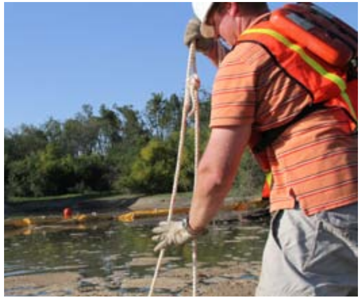
Step 9: Set the anchor for maximum loadlock by pulling vertically on the rope with a substantial amount of force. This will shift the anchor into position for full stability.
