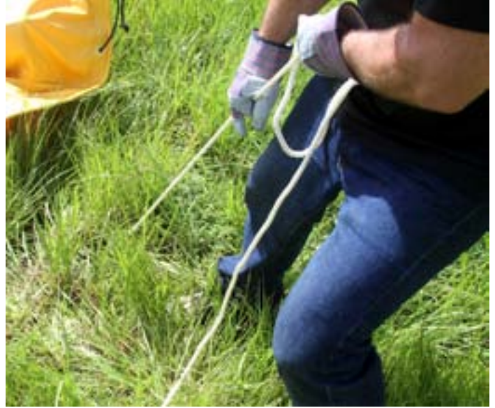
Step 7: Set the anchor for maximum loadlock by pulling vertically on the rope with a substantial amount of force. This will shift the anchor into position for full stability.
