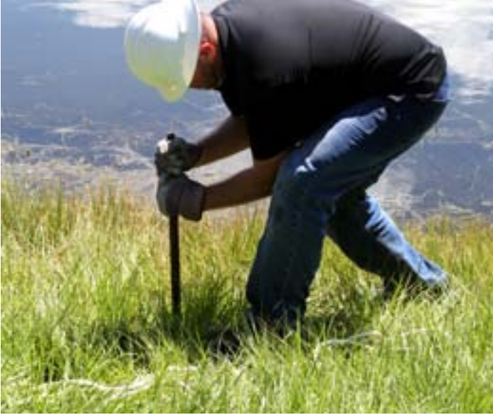
Step 6: Twist the rod so it loosens from the anchor. Pull out the rod once it is completely loose.
