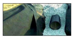
Stormwater runoff disturbs soil near french drains, during rip rap installation, and asphalt overlay. **Geotextiles** are used as a means of separation, stabilization, filtration, and slope protection, to control soil particles as they are displaced.
