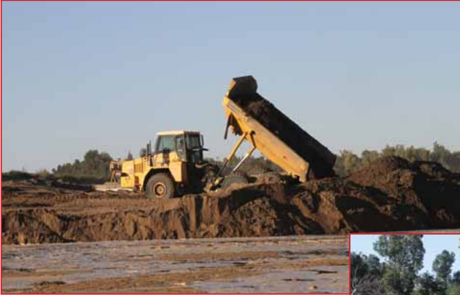
Top: Filling of the scour hole. Right: Installed silt curtains help prevent spreading of materials during scour hole filling. Images courtesy of Granite Environmental, Inc.
