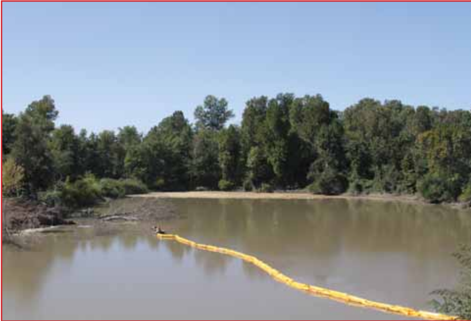
Silt curtain being deployed. Image courtesy of Granite Environmental, Inc.
