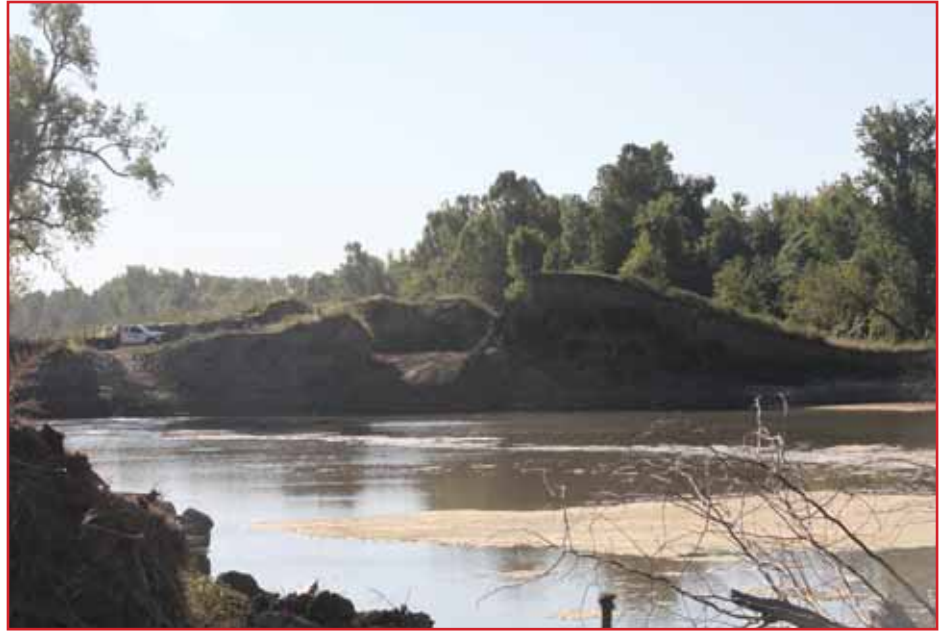
Location prior to installation of the turbidity curtain.
