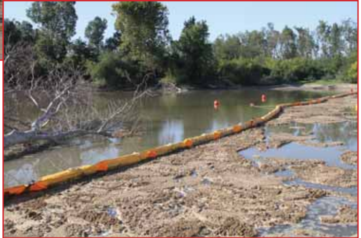
Top: Filling of the scour hole. Right: Installed silt curtains help prevent spreading of materials during scour hole filling. Images courtesy of Granite Environmental, Inc.
